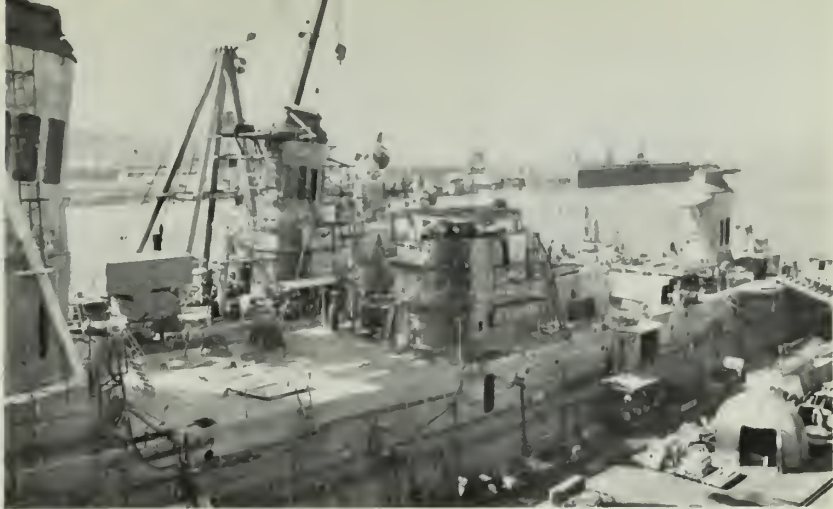
(16) Work begins on superstructure
